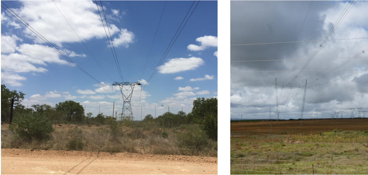
Figure 11: Example of a self-supporting tower (left). Example of a cross-rope suspension tower (right).
